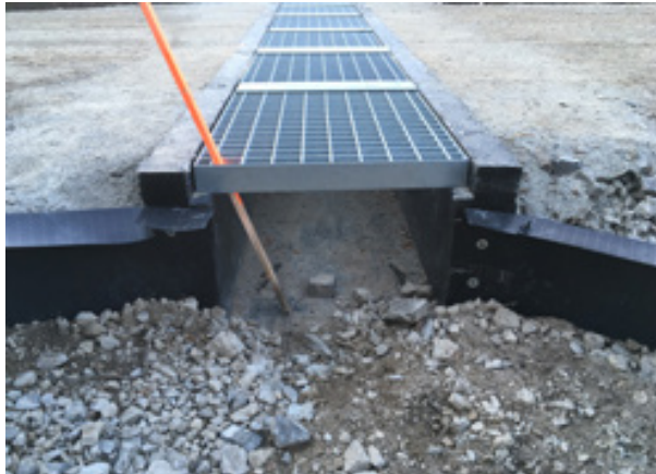
Many types of culverts can be utilized and often are constructed specifically as ecopassages.
